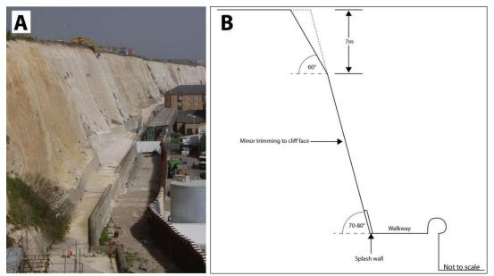
Figure 36: Cliff trimming of the chalk cliffs in Brighton Marina (A) Image of work being undertaken (University of Sussex, 2013) and (B) schematic showing detail of work (High-Point Rendel, 2002; 2006).
