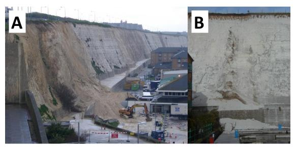
Figure 38: Cliff failures in Brighton Marina during the winter of 2000/2001 (A) Black Rock affecting commercial properties (B) in Newhaven Chalk which almost hit the residential properties. (Image source: University of Sussex, 2013).
