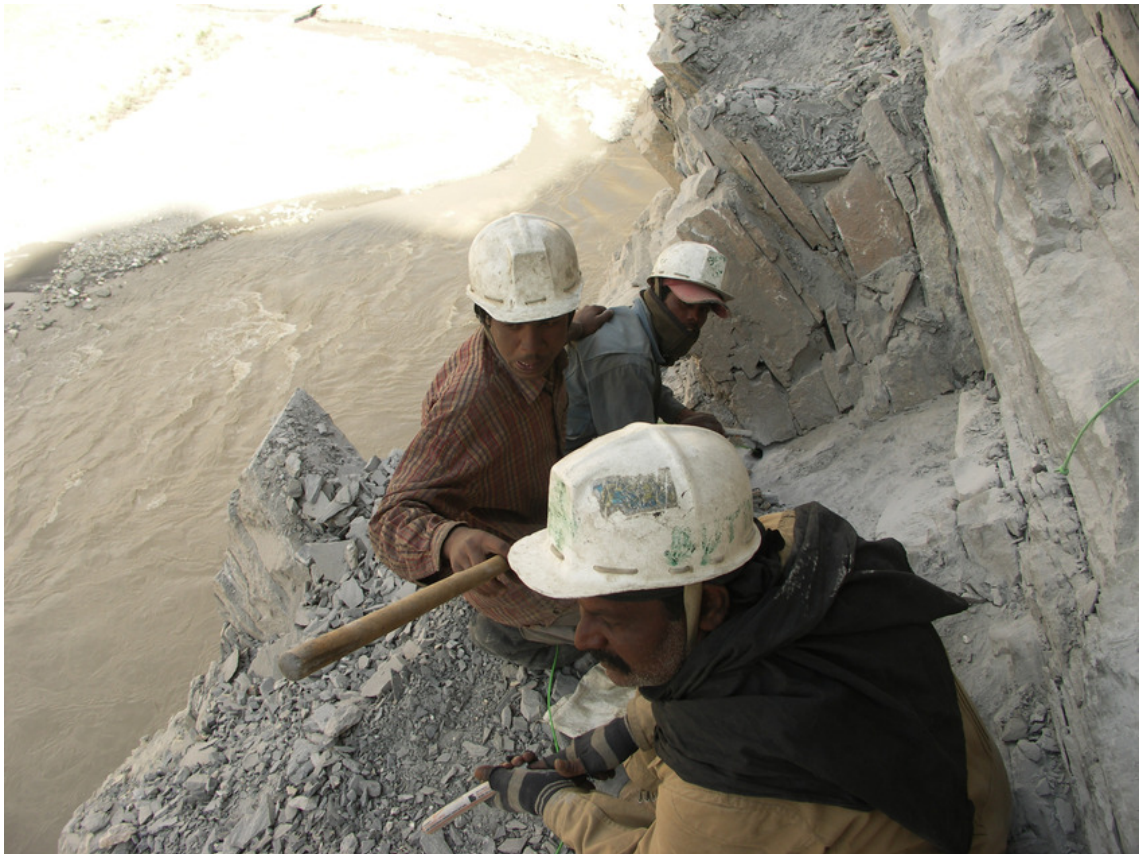
6.10. Filling holes with explosives on Lamaguru Mountain (June 2007)
