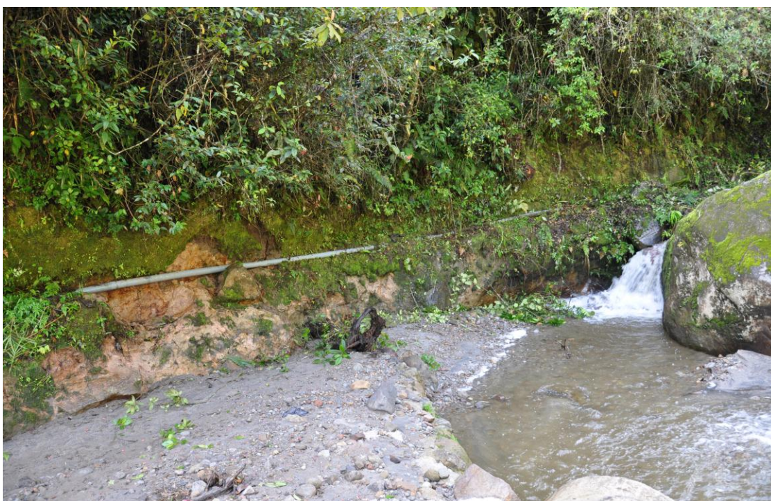
Figure 5.3. Main pipe that takes water from the spring to the collection tank
