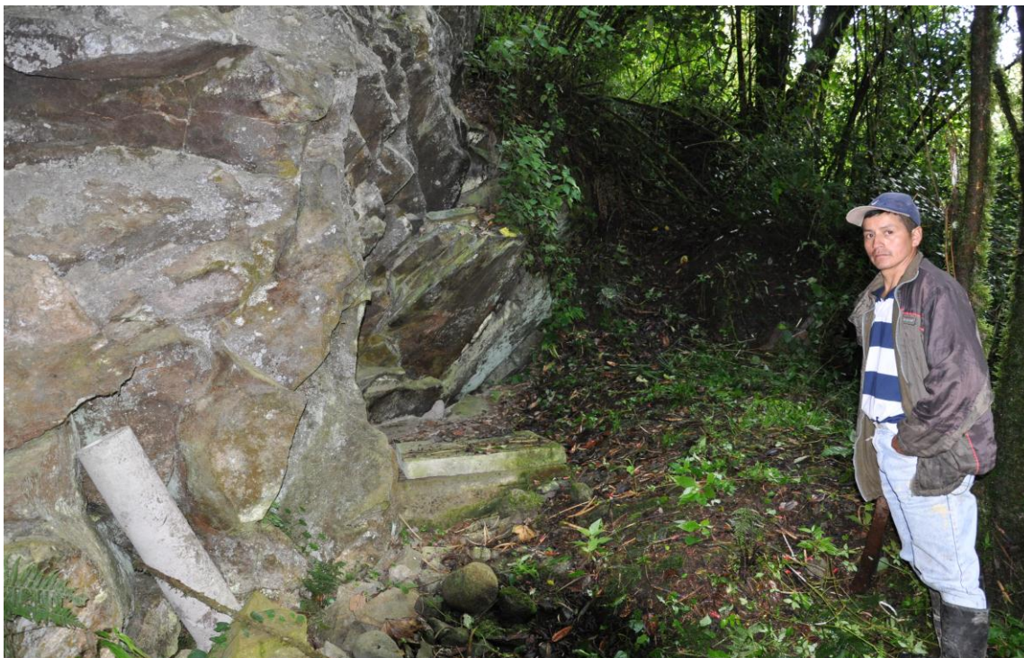
Figure 5.3. Main pipe that takes water from the spring to the collection tank
