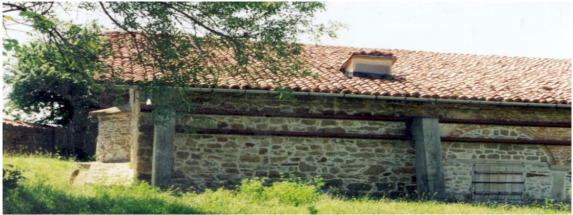
Fig.33: Supporting system of concrete buttresses on the south façade of the Church of the Nativity of Christ.
