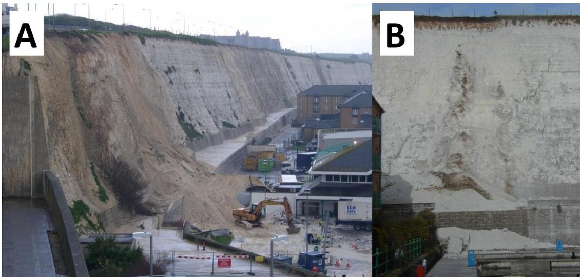
Figure 38: Cliff failures in Brighton Marina during the winter of 2000/2001 (A) Black Rock affecting commercial properties (B) in Newhaven Chalk which almost hit the residential properties. (Image source: University of Sussex, 2013).
