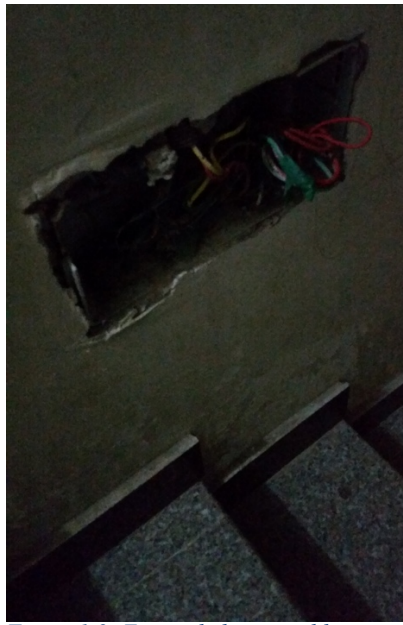
Figure 1.9: Exposed electric cables
