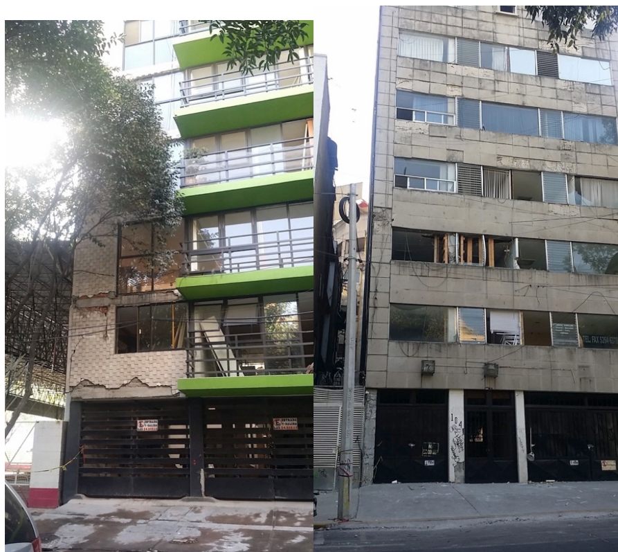
Figure 4.4: Buildings that show structural damage but remains standing in the neighbourhood La Condesa
