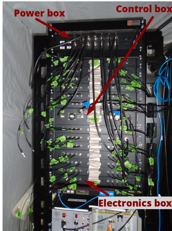
Figure 4.2: A photo of the TELLIE rack in the DCR. The power box, control box and an electronics housing box are identified.
